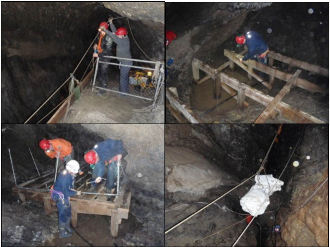
Plate 6: Dismantling and removing the holding tank, June 2010. Photos: Rolan Eberhard
